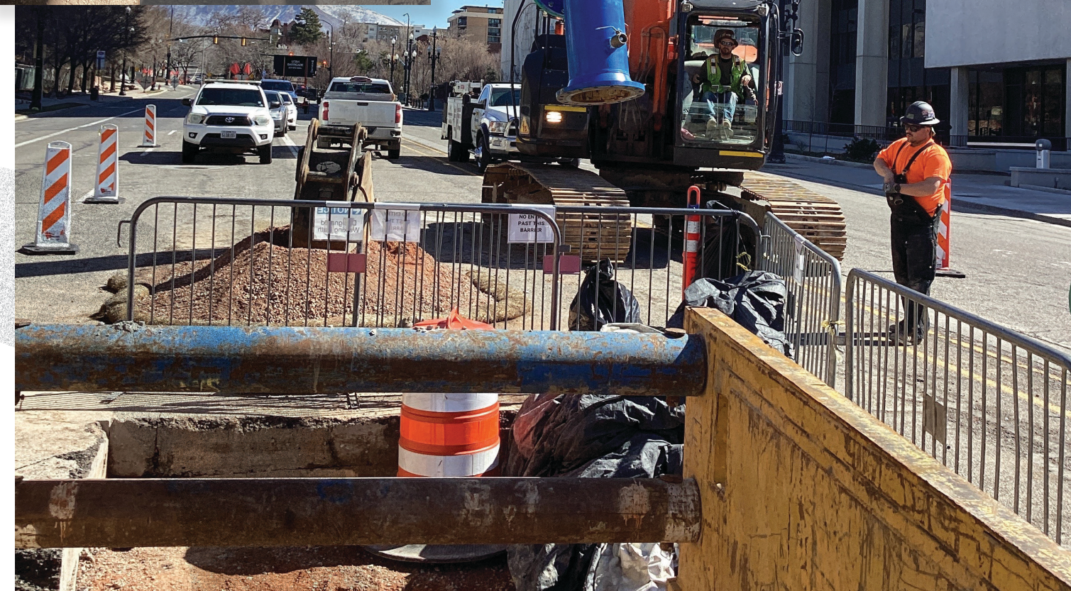
Installing a new 24" sewer main in North Temple
